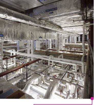
Fresh air: A labyrinth of ducts guides air in the lab through banks of powerful filters, each of which removes more than 99 percent of particles larger than 0.0003 mm. Staff say air leaves the building cleaner than it arrives.
